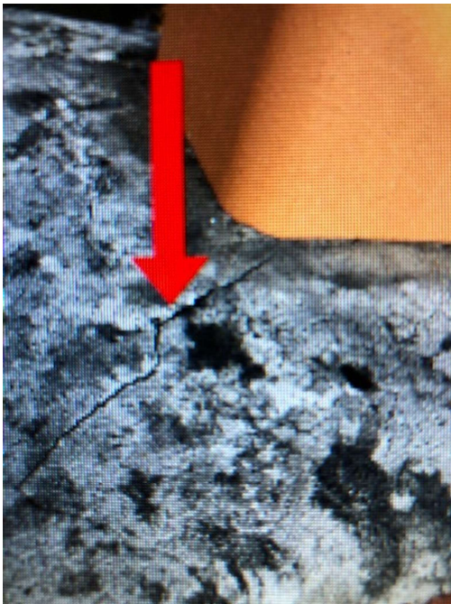
Cracked chimney crown.
