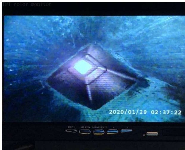
Interior of flue assessed with camera – appears satisfactory.
