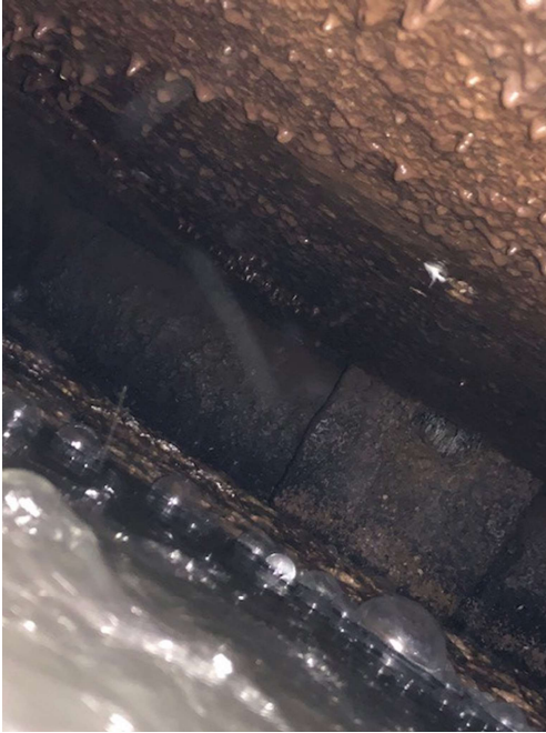
Outlet baffle intact and satisfactory.
